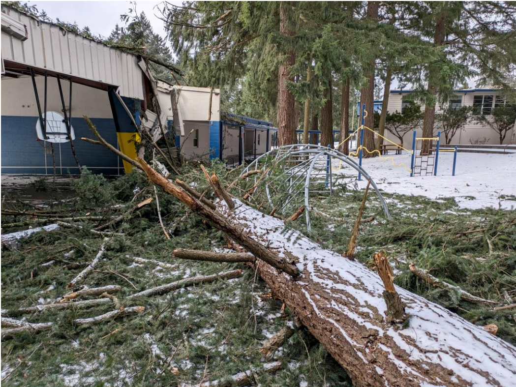
Portland Public Schools suffer damage during historic ice storm Credit: OPB
