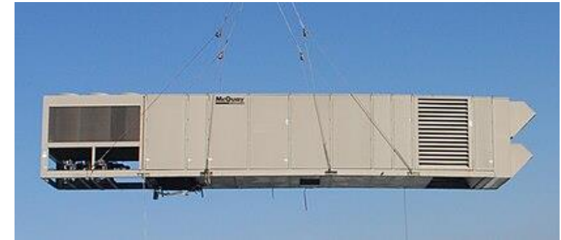
Air Handling Units (AHUs)
