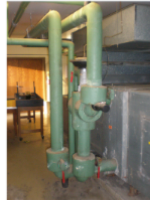
ECM 9b-1 – Rockingham High School Chilled Water Pipe Insulation
