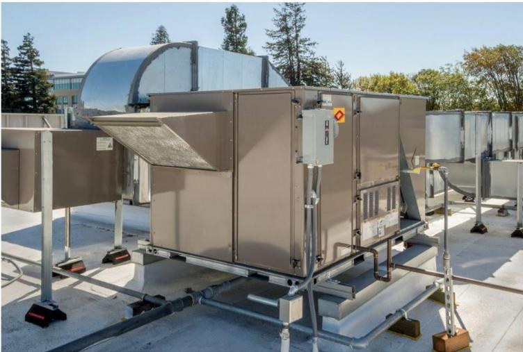
The Rooftop unit (RTU) replacement package includes a high-efficiency RTU, advanced controls based on ASHRAE Guideline 36, and energy monitoring. Optionally and where appropriate, the package also includes window films and cool roofs to reduce the RTU load and size.
